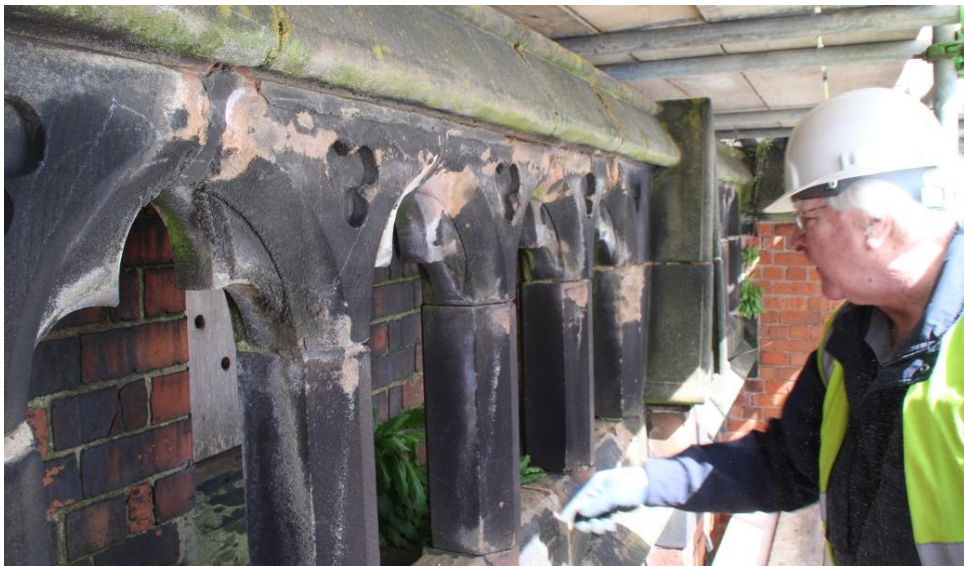
Fred Tandy, our Structural Engineer, inspects the sandstone balustrade at the west end from the scaffolding. This was subsequently taken apart, repaired and reinstated.
