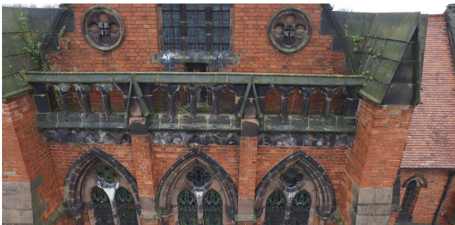
The west end: UAV view of high-level stonework in poor condition and the tops of the three sections of the Great West Window. (Aerial Video TV).
