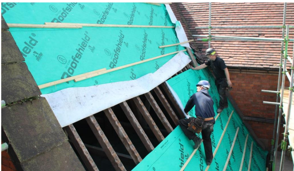
Two of HCR's roofers applying a breathable geotextile membrane to a section of transept roof before retiling can take place.
