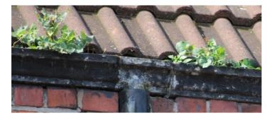
Gutters: this plant growth is a clear sign that the gutters have gone some time since they were cleared out. Skimping on gutter maintenance is a false economy! You should also check the hopper heads which act as a funnel to prevent overflows of water between the gutters and downspouts. Again plant growth is a clear sign of a blockage which has been left unattended for too long.
