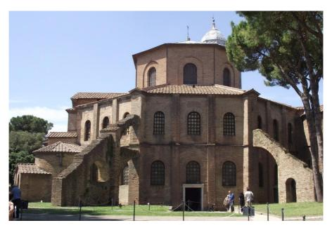
Architecturally, the Basilica is constructed to an octagonal plan. The building combines elements of Roman and Byzantine architectural styles. The brickwork is typically Byzantine with narrow bricks and thick mortar joints but the doorways and dome are distinctly Roman.
