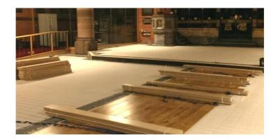
Good progress is being made at **St. Dunstan's**, Edge Hill (1889 by Aldridge & Deacon, Grade II\* Listed). This photo, taken on March 4<sup>th</sup>, shows the first new engineered oak floorboards laid atop the underfloor heating system which was handed over on February 27<sup>th</sup>. St. Dunstan's will be re-opened on Maundy Thursday at a special service with Rev. Richard Giles in attendance.
